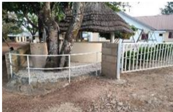
Figure 12: Iron work in play areas created from recycled plumbing pipes after replacement with new PVC pipes
